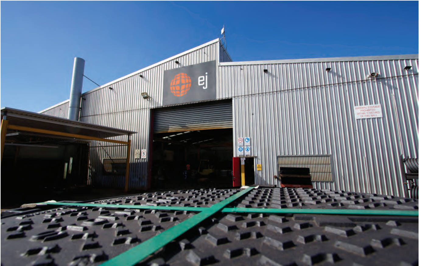
Queensland Factory, Brisbane, Australia.
